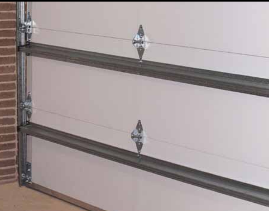
Thermal barrier joints seal off the gaps between each panel.
